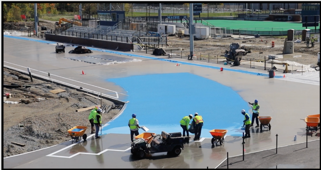
Construction being done on the new track and field at UMaine on Sept. 26. PHOTO BY OBIE CASPERSON
