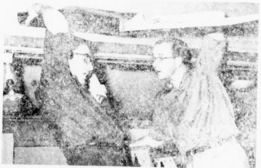
Lawrence Eaton and Richard Lunt attempt to hang a checkerboard ceiling from atop a rickety ladder.
