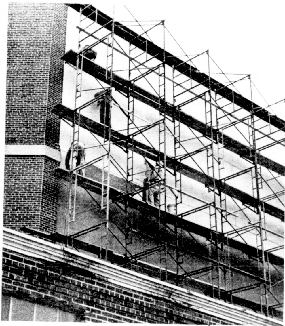
Not just hanging around, but making some repairs Wednesday at the Memorial Gym Fieldhouse. [photo by Lloyd Rees]
