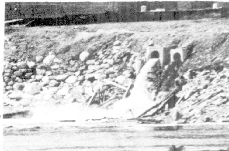
Industrial waste contributing to Maine's water pollution problem.
